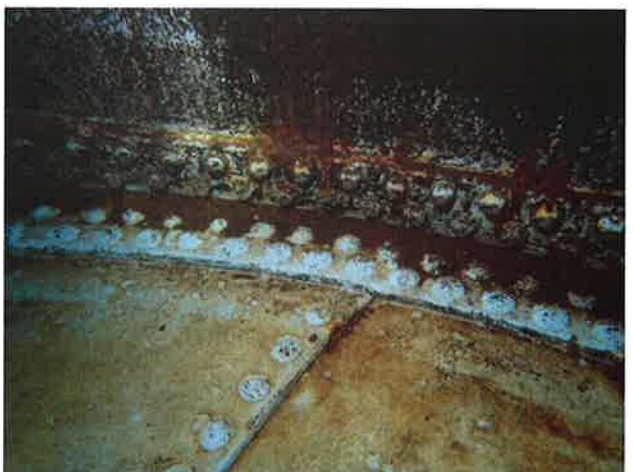
54 Floor With Mild Staining
