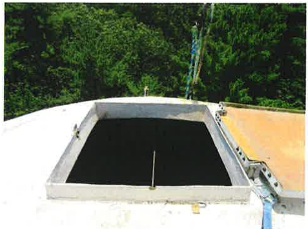
44 Open Access Hatch
