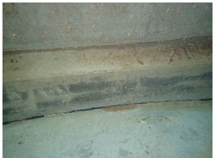
72 Interior Concrete Curb
