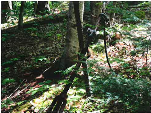
25 Support Cable Secured To A Turn Buckle
