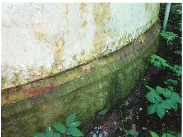
30 Granite Block And Stone Foundation
