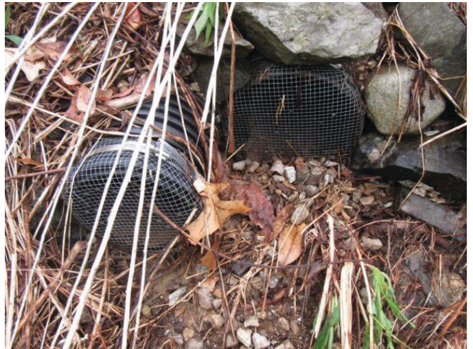
16 Secure Overflow Pipe Screen
