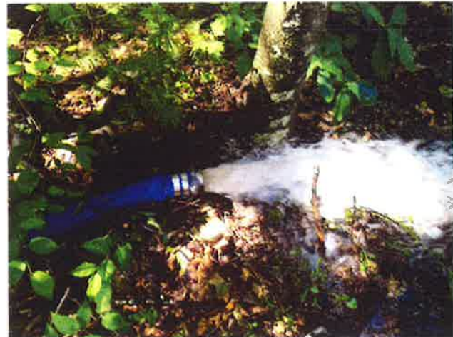
90 Discharge During Cleaning
