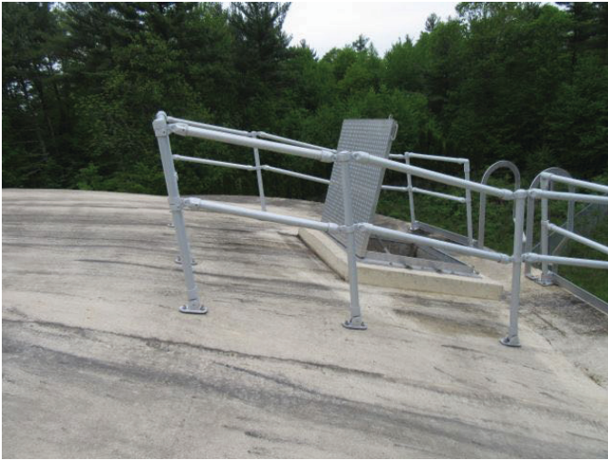
25 Secure Safety Railing
