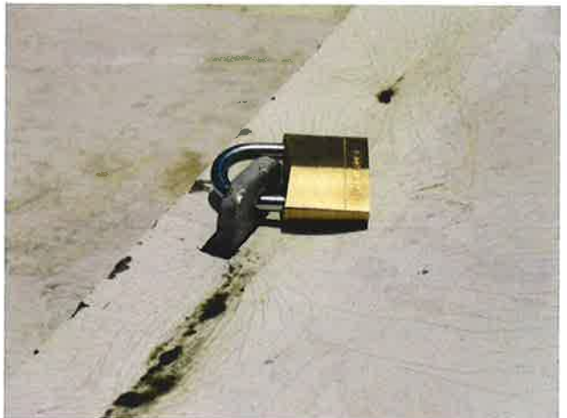
46 Secure Access Hatch
