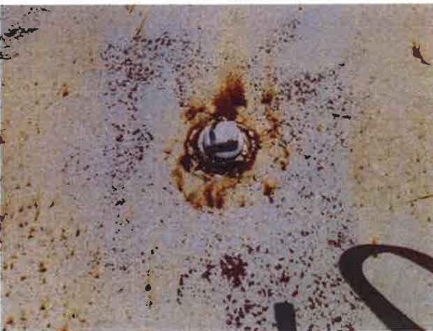
35 Secure Roof Dome Rigging Hole
