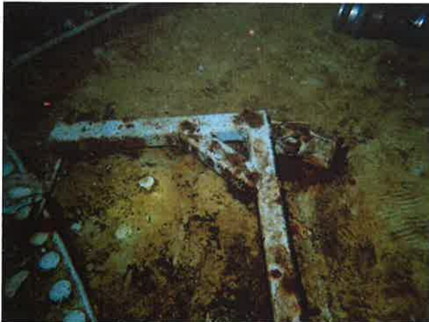
57 Manway Steel Support Laying On The Tank Floor
