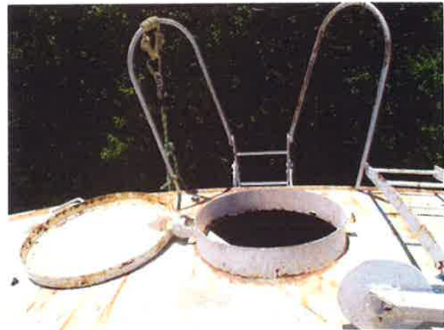
40 Open Access Hatch
