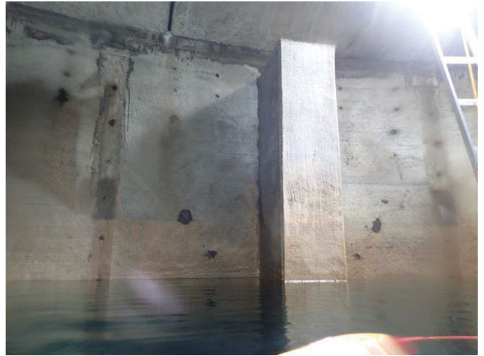
86 Concrete Overflow Box
