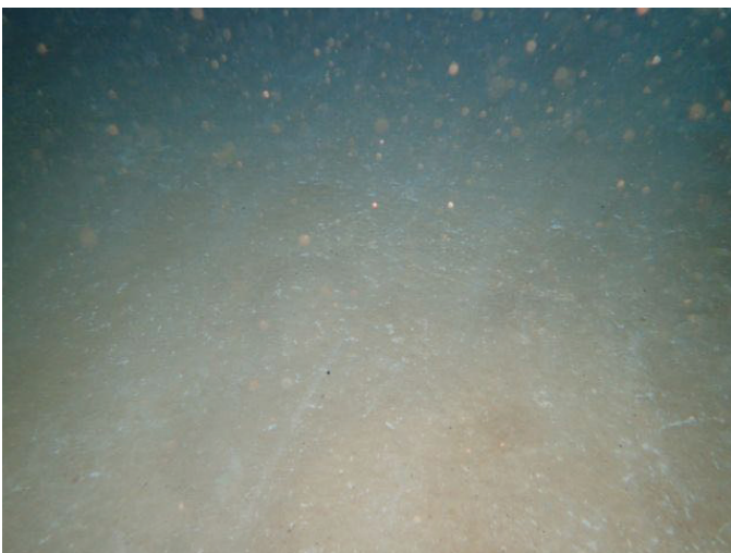
41 Floor With Mild Staining
