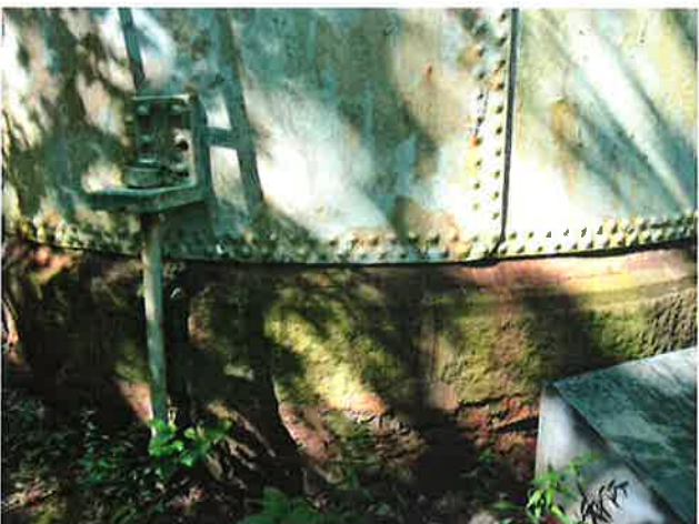
29 Granite Block And Stone Foundation
