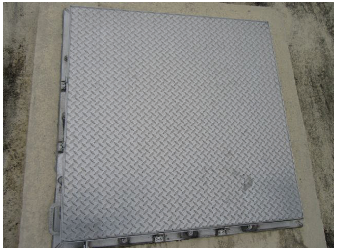
30 Closed Access Hatch
