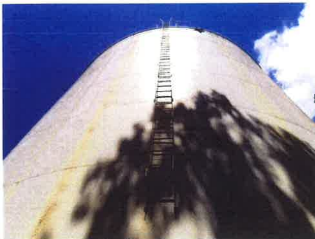
23 Roof Access Ladder
