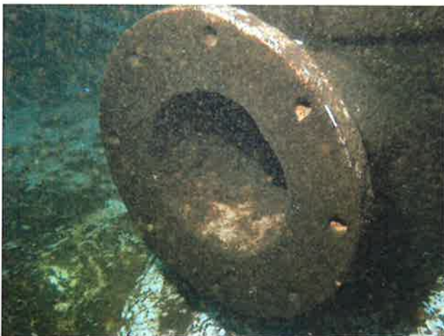
59 Inlet/Outlet Pipe With 12" Inside Diameter Penetrations
