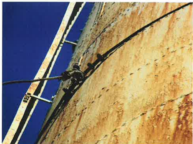
22 Exterior Wall With A Support Cable
