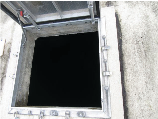
29 Open Access Hatch
