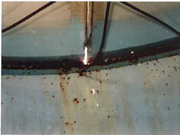
79 Overhead With Daylight Showing Through The Panel Joints
