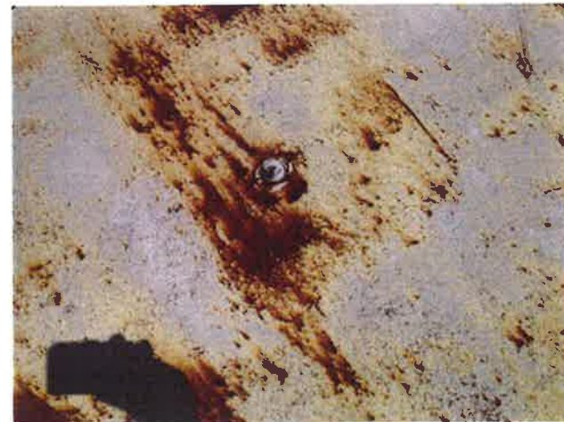
36 Secure Roof Dome Rigging Hole
