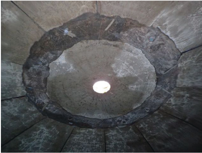
79 Overhead With A Vent Penetration
