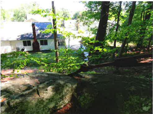
27 Support Cable Turn Buckle Secured To A Pad Eye Drilled Into A Large Granite Boulder
