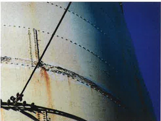
23 Exterior Wall With A Support Cable
