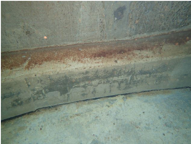
73 Interior Concrete Curb
