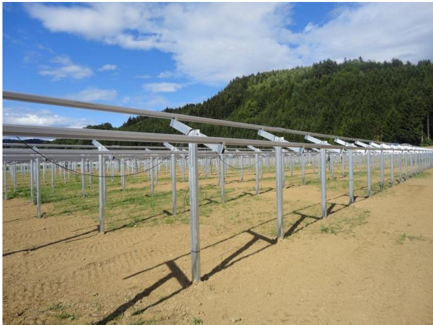
Racking equipment – prior to panel installation.
