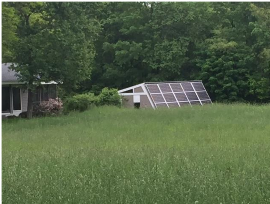
Residential Ground mounted system.
