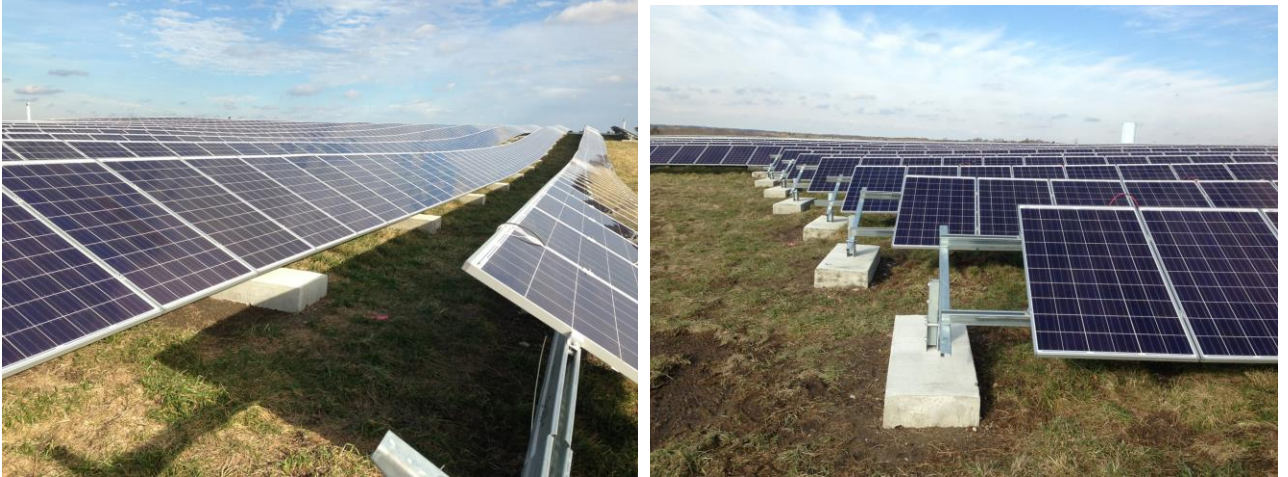
Ballasted system, showing distance between rows and the ballast blocks.
